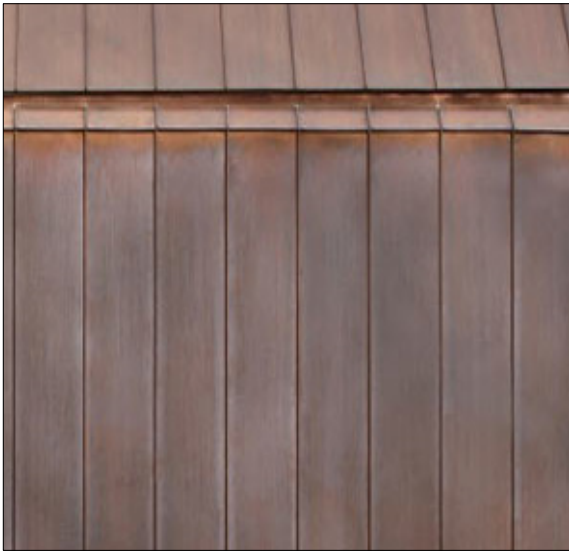
PRE-WEATHERED STANDING SEAM COPPER ROOF 350-450MM WIDTH
