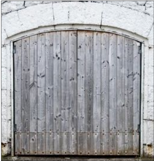
BOATSHED TIMBER DOOR
