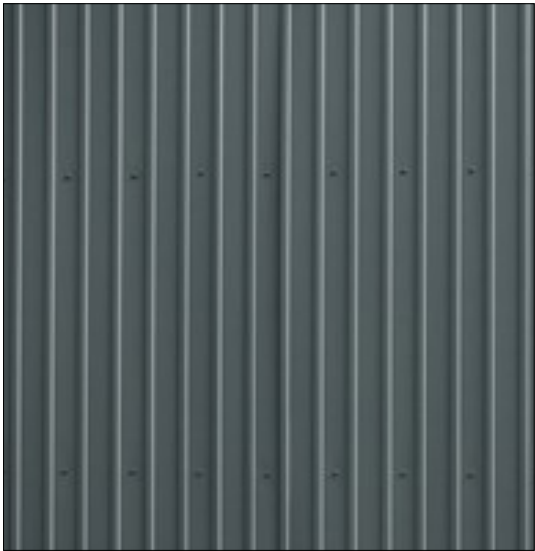
EXISTING METAL ROOF
