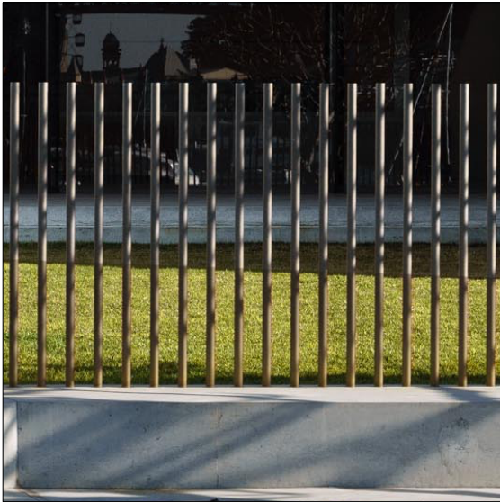
CONCRETE CAPPING + STEEL BALUSTRADE
