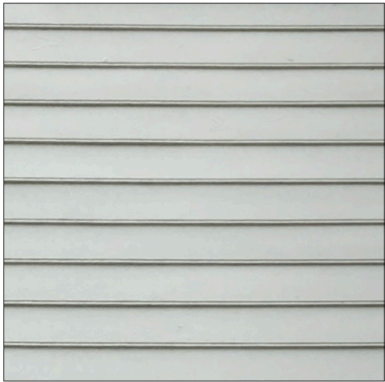
EXISTING WEATHERBOARD CLADDING
